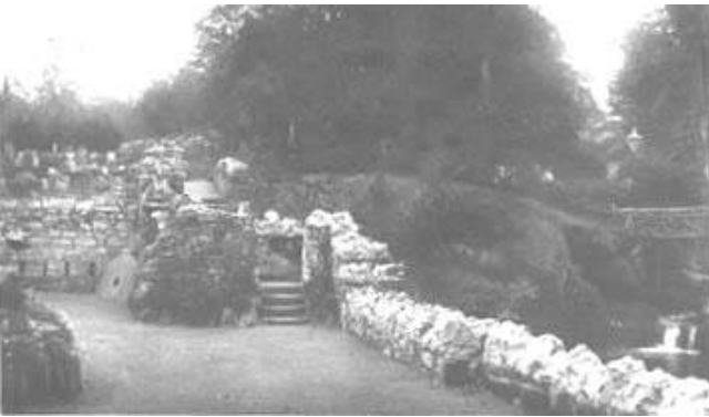
Remains of Millig Mill in Hermitage Park, Helensburgh
