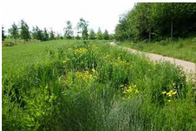
A swale in the North Park, part of the SUDS design that helps to slow the flow of water into the River Lee; as well as being a natural form of flood defence, the swales also function as biodiversity habitat.
